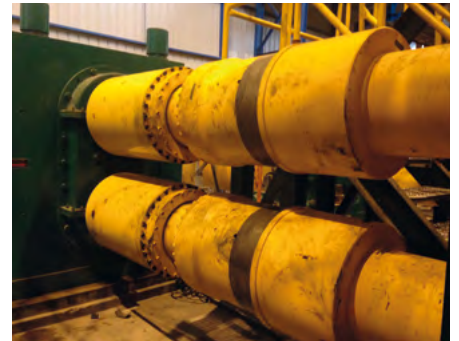
Continuous strip production spindles on site
